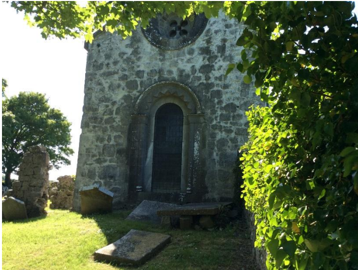
Plate 13-1: Romanesque doorway of church at Rahan Demesne.
