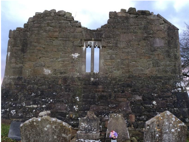
Plate 13-5: East gable of church OF015-004003, looking W.
